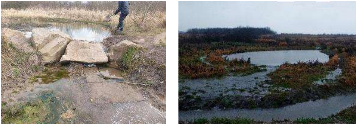
Figure 20 Leaky dams: volunteer help & storm water retention (Source Bickershaw Project Facebook)
