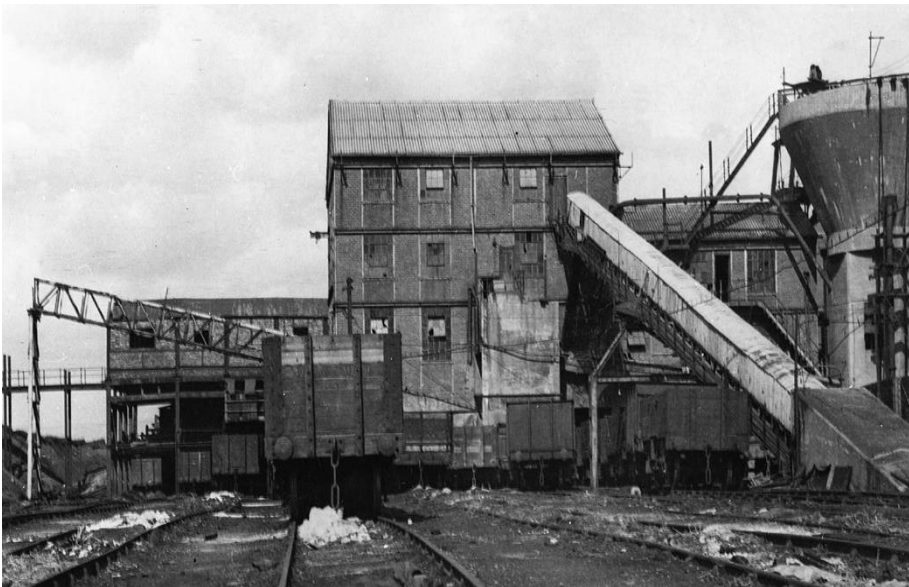
Screens at Garswood Hall Colliery
