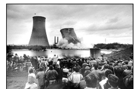
Westwood Power Station
